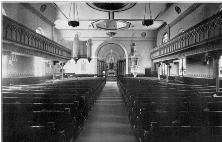
INTERIOR OF 1929 CHURCH
